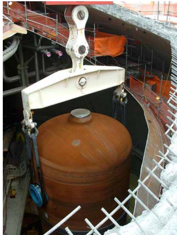
Fig. 24. Rigging SGR into containment building.
