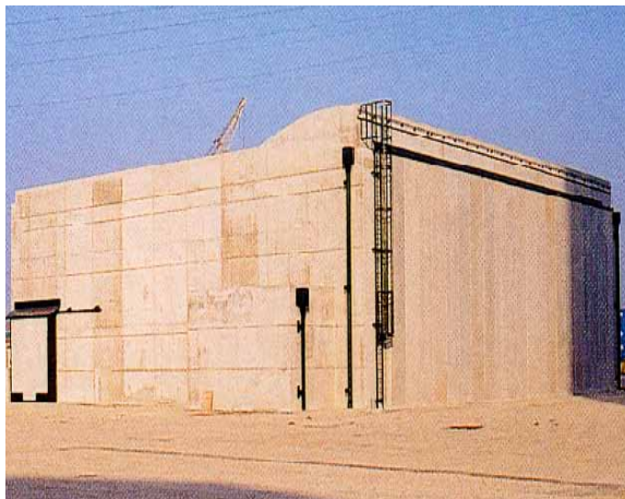
FIG. 59. Example of decommissioned SG mausoleum in France.
