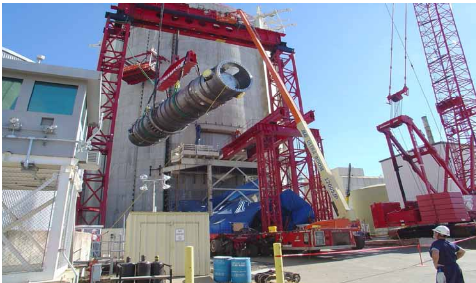
FIG. 21. SG rigging outside containment.
