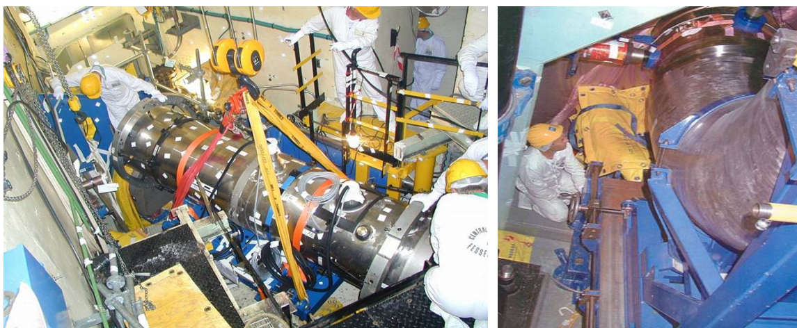
FIG. 42. Replacement RCL pipe.
