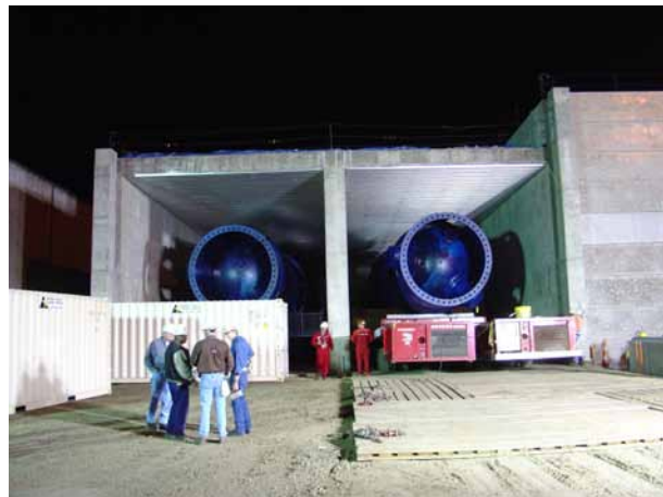
FIG. 60. Example of decommissioned SG mausoleum in the USA.
