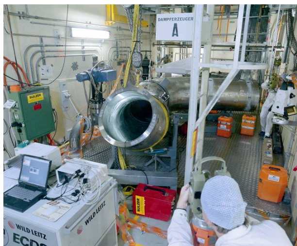
FIG. 41. New RCL pipe spool, welding already completed on-site, during 3-D topometry inspection ready for transportation to its welding position.
