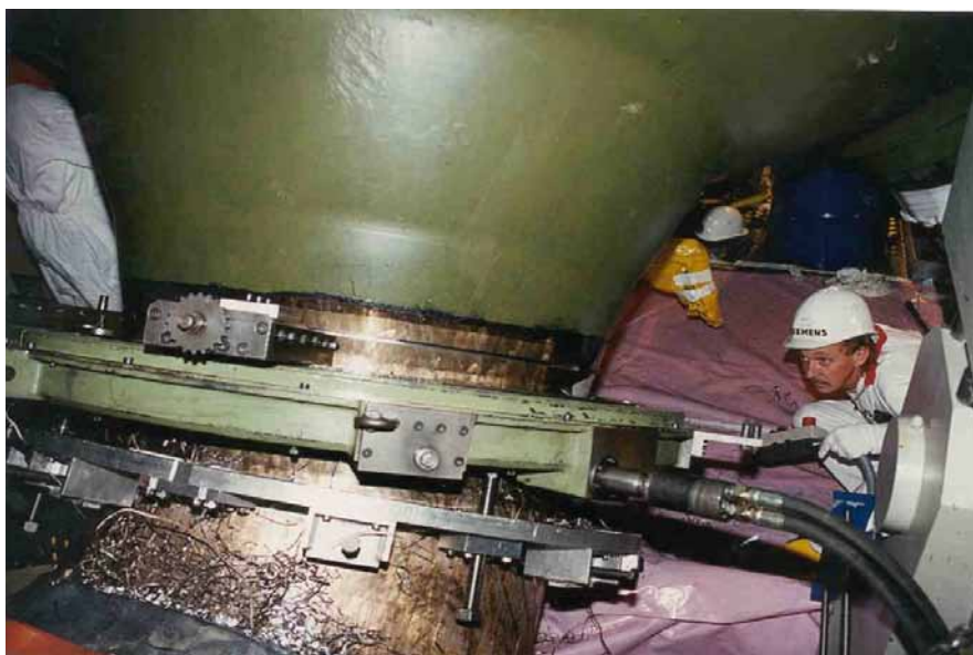
FIG. 16. Pre-cutting of the reactor coolant piping.
